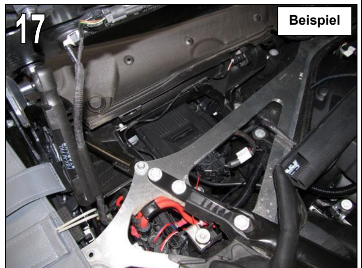
Fig. 17 Attach the AC Schnitzer control unit to the fuse box using the bracket supplied, inc. double-sided adhesives strips.
